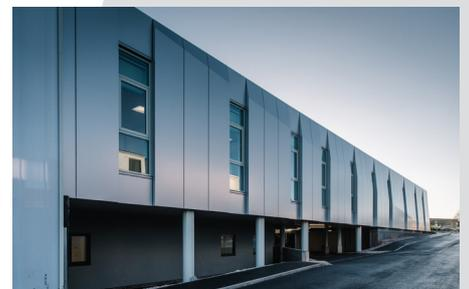
“ One of the building's stand out features is the side elevation which incorporates an innovative 'architectural crease' design, created using the PVDF finish from the Alucobond panels. ”
